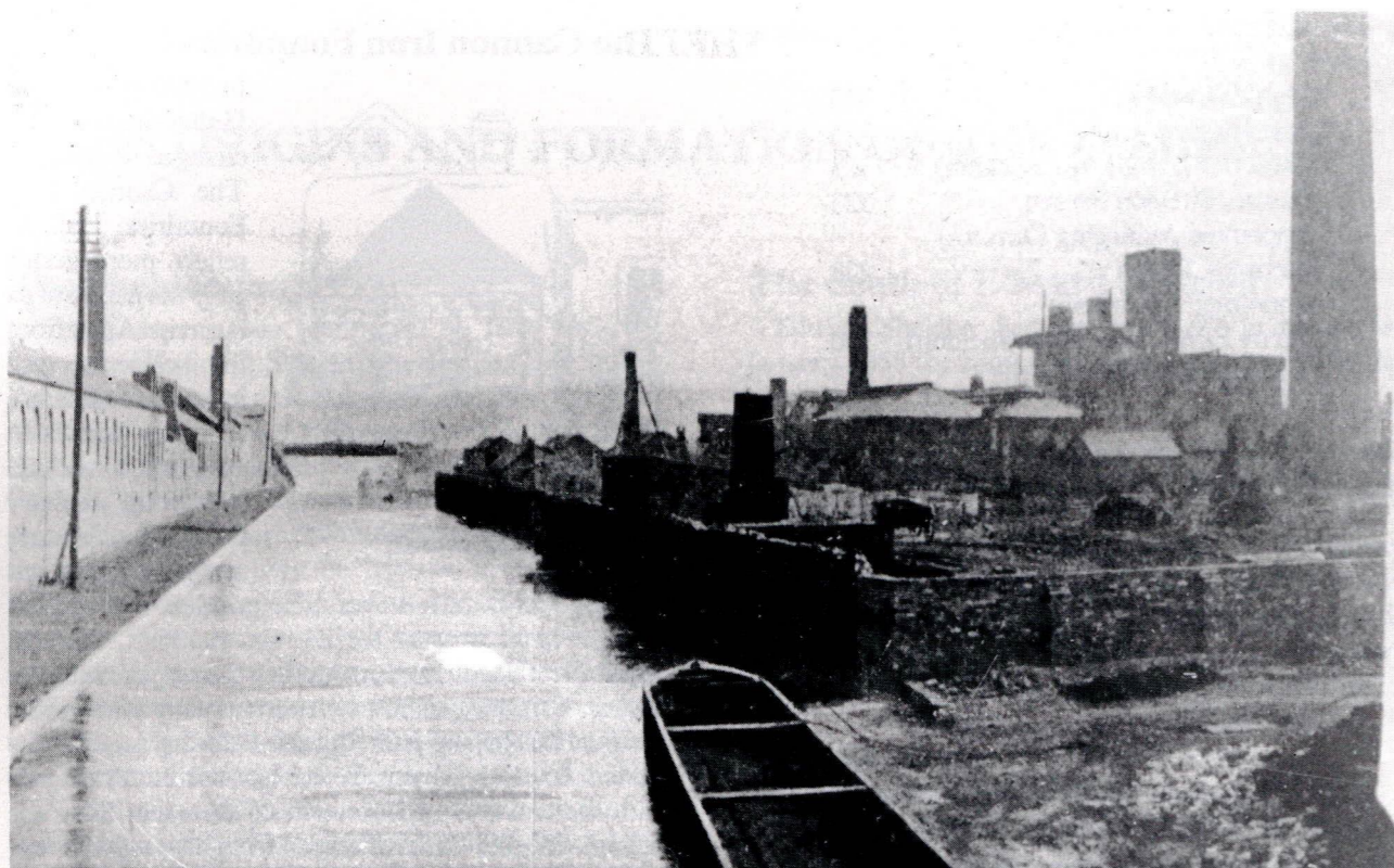
The Birmingham to Wolverhampton Canal, looking towards Coseley Tunnel, that divided the Cannon Iron Foundry on the left from the Priorfields Iron works (that supplied pig iron to Cannon) on the right.
