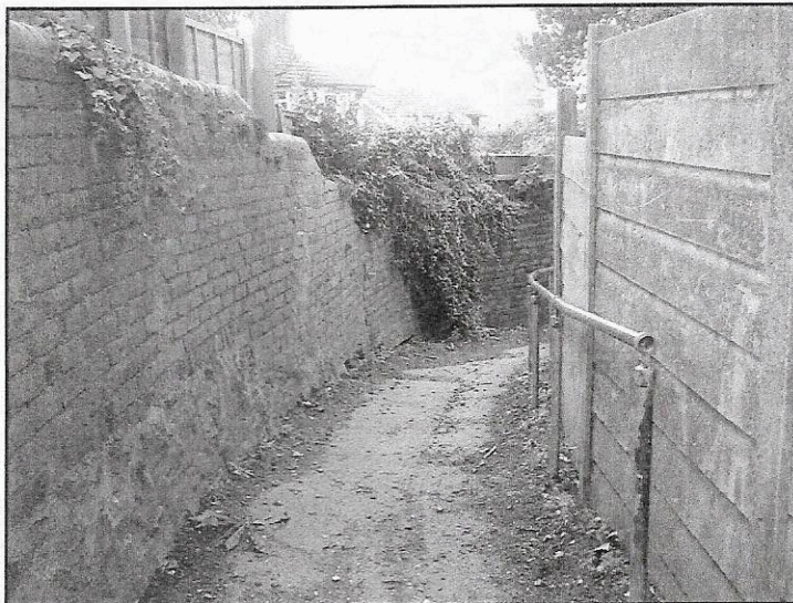
The Gully in 2004. The old Victorian Vicarage wall on the left set on exposed sandstone, and the modern concrete hospital wall to the right. However both are very new in comparison to the actual track way they define.
