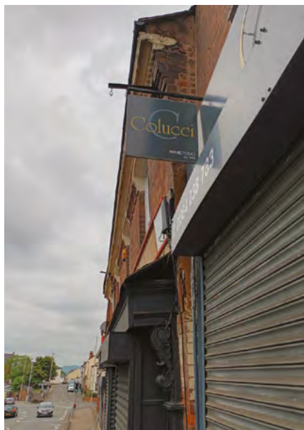
THE SAMPSON AND LION BUILDING FRONTAGE LEANING SOME TWO FEET TOWARDS THE ROAD, SINCE COMPENSATION WAS USED TO STABILISE RATHER THAN DEMOLISH.
