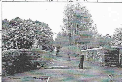
Seven Dwellings Bridge. Enoch and Caroline took this route heading for the Birch Tree after leaving Annie Westwood.
