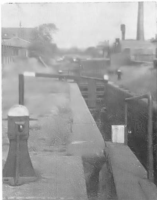
View from Wolverhampton Street, Walsall, showing lock no. 6. This is unusual, in that it has mitre bottom gates as opposed to single gates on the other seven.
